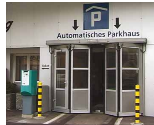
Skyline L-Park in operation: the parking procedure with conveyor belts at an installation in Switzerland
